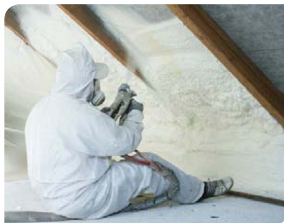
Above: A worker spraying polyurethane foam insulation in a loft space.
