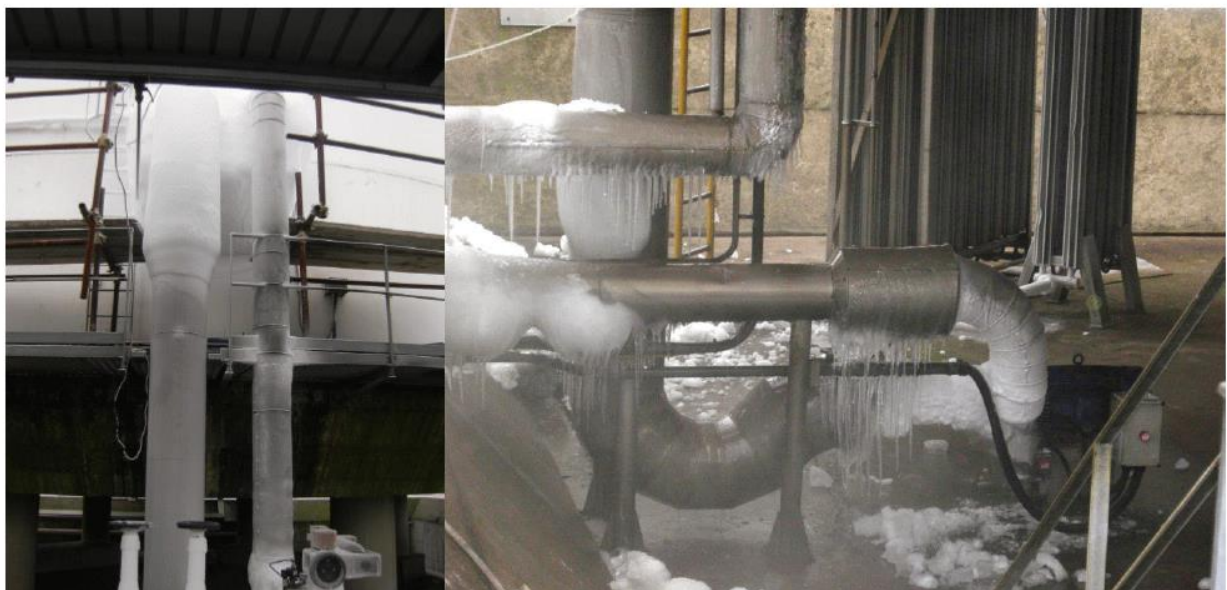
Broken vapour barriers and insufficient insulation caused ice to form around these pipes causing both process control and structural problems
