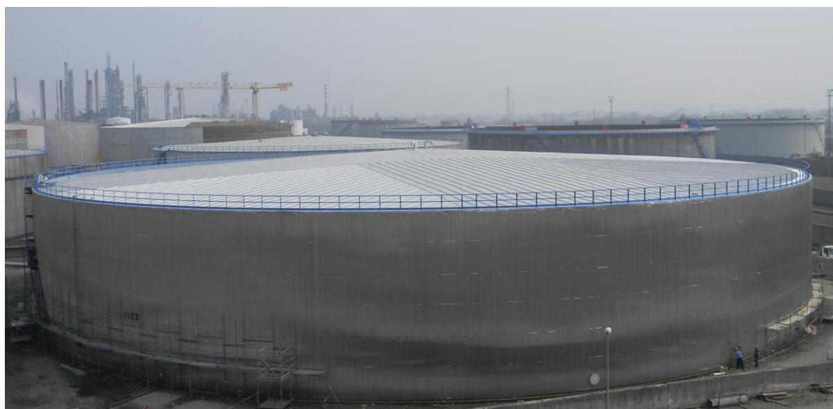
AFTER: The tank roof newly insulated with a 30 mm insulation solution and long-lasting corrosion protection
