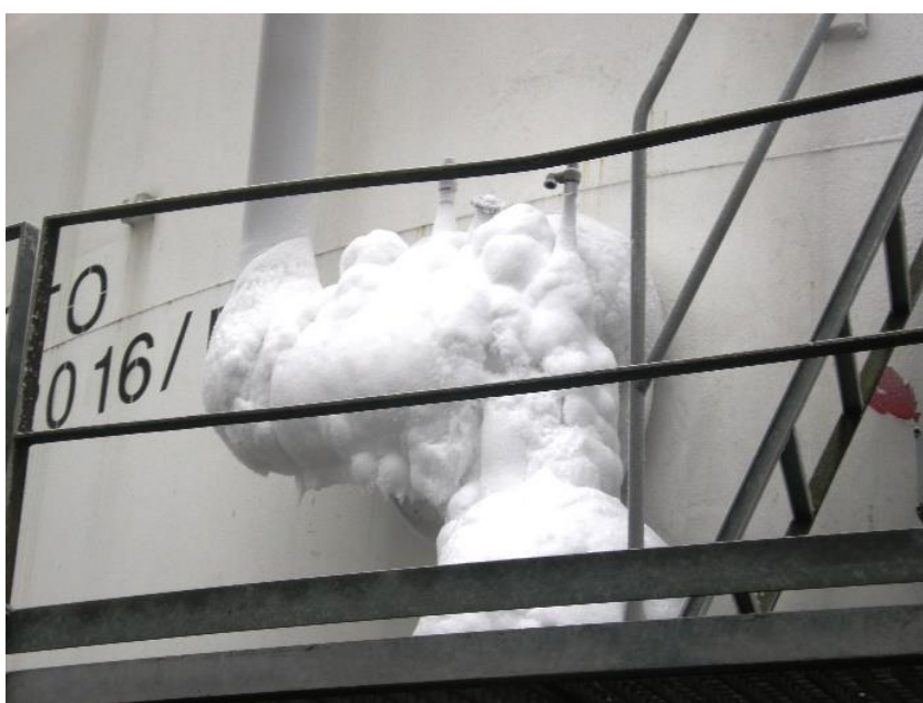
Valve fully covered with ice can no longer be operated
