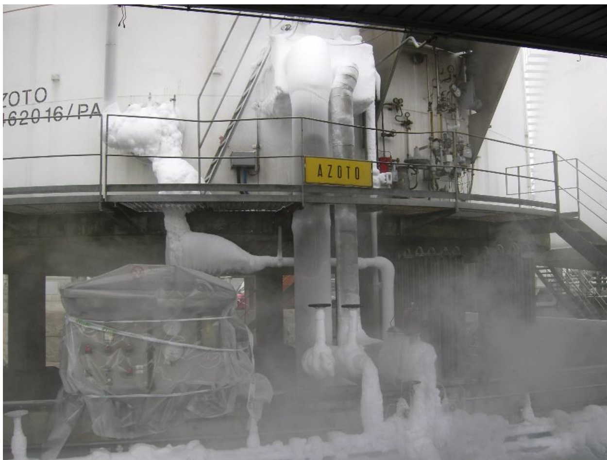
Control panel “protected” with plastic sheeting from the dripping condensation water. Extensive ice formation on pipes and valves
