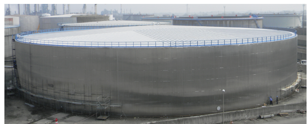
AFTER. The tank roof newly insulated with a 30 mm insulation solution and long lasting corrosion protection.
