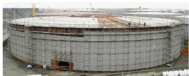
BEFORE. An aged oil storage tank in a refinery had a heavily corroded roof and urgently needed repair.
